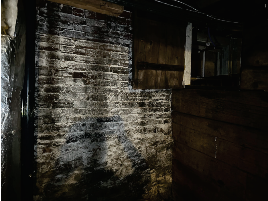
Interior view of Southeast perimeter wall
