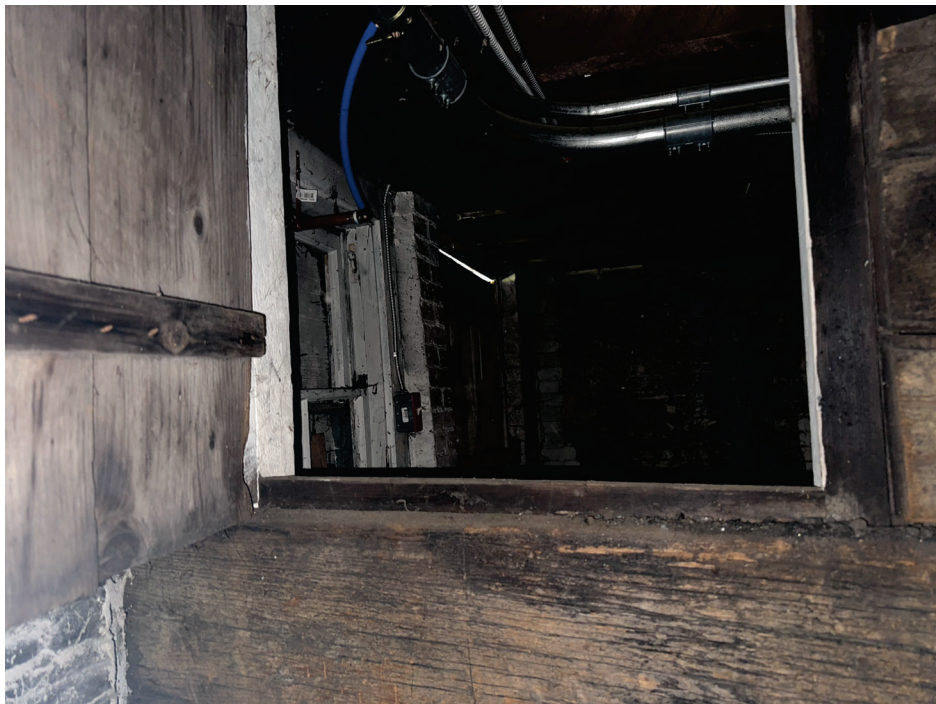
Floor joists along Southeast perimeter wall
