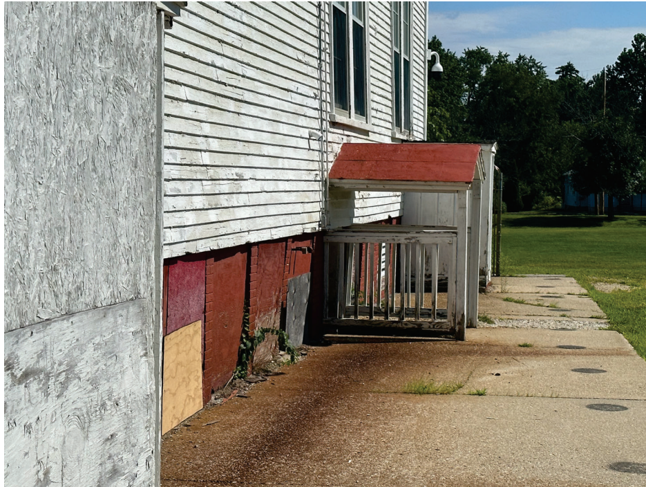
Southeast perimeter wall
